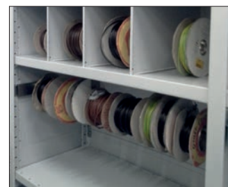
Cable reel storage - Reels are located on a central rail allowing easy dispensing of cable.
